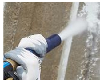
Concrete Surface Prep
