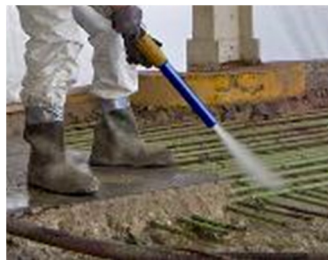
Concrete Repair & Restoration
