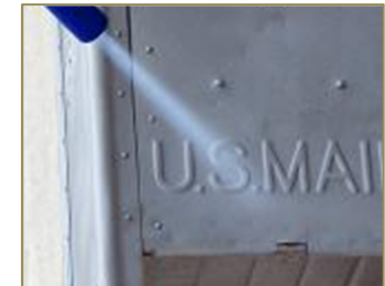
Steel Surface Prep
